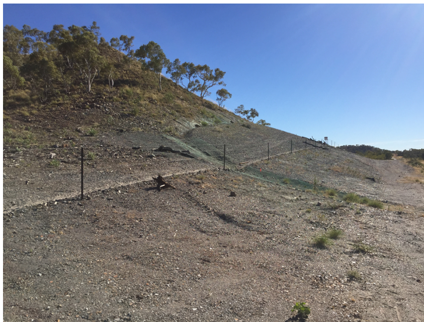
Figure 8. Photograph of KP 618 showing re-profiling on hillside
