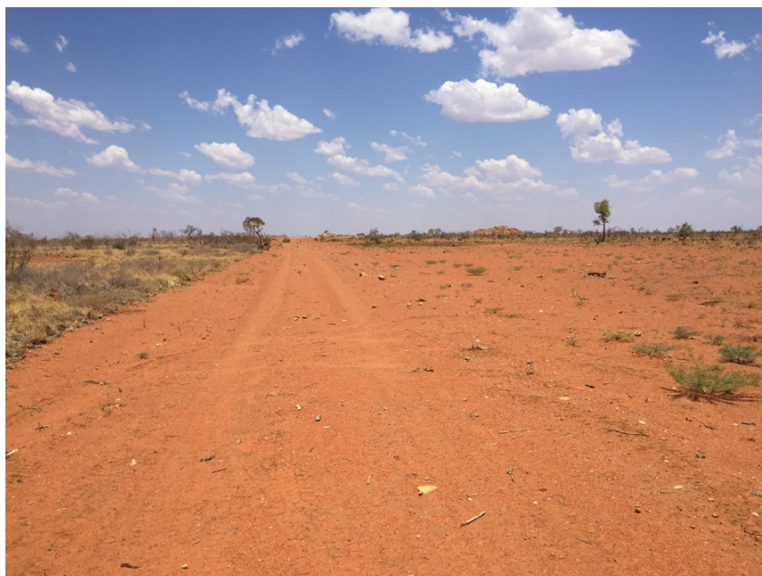
Figure 12. Photograph of ROW (to the right of the access track) showing little vegetation growth (KP 32)
