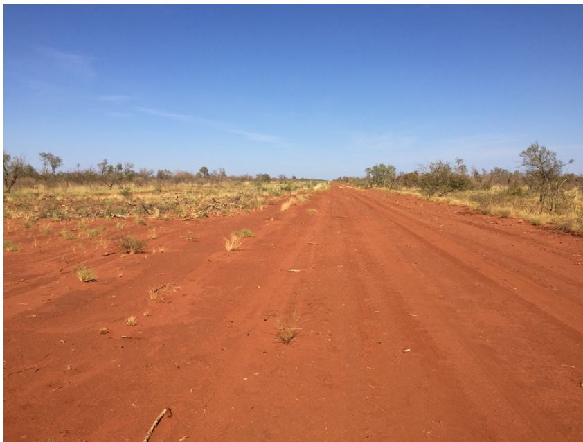
Figure 14. Photograph of ROW at KP 91
