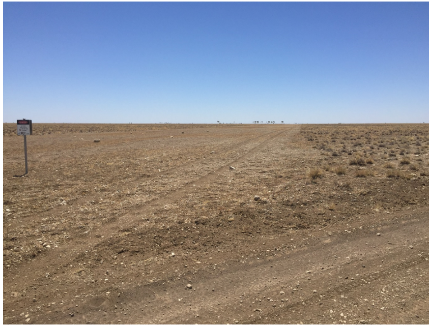
Figure 7. Photograph of KP 468.4 showing re-profiling
