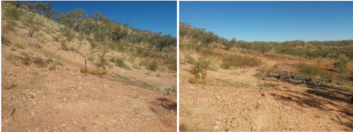
Figure 15 Water diversion trench on slope at ~KP 620
