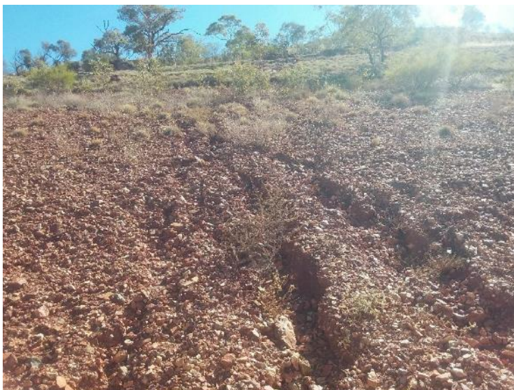
Figure 16 Erosion Gully forming down slope at ~KP620
