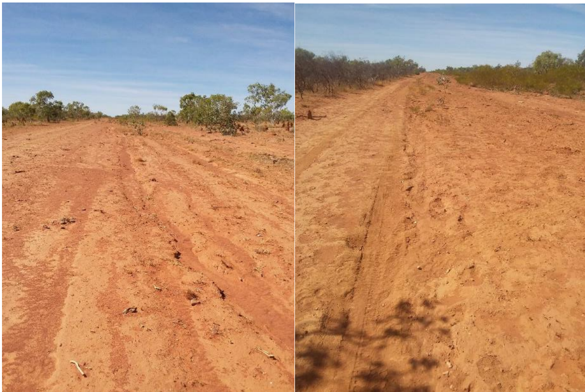
Figure 11: Minor shallow rill erosion (KP 24.7 & KP 27.4)
