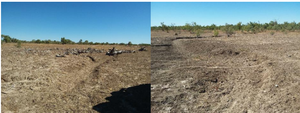
Figure 13 Moderate Extensive Erosion (KP 410.3)
