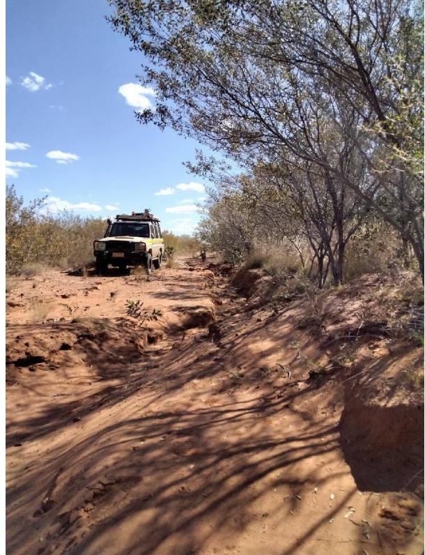
Figure 11. Significant erosion with over 700mm deep gully erosion KP 267.5
