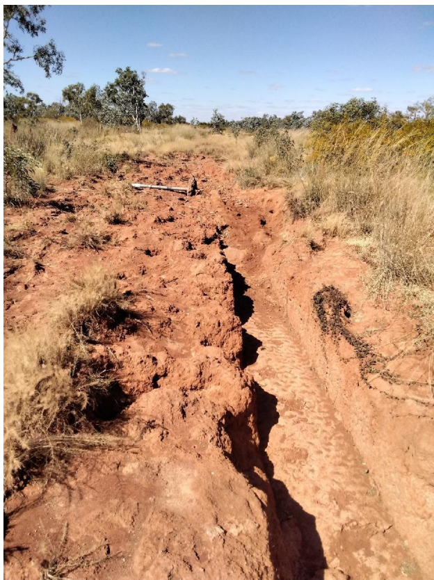
Figure 21. Significant subsidence up to a metre deep at KP 25 where runoff follows the pipeline trench.
