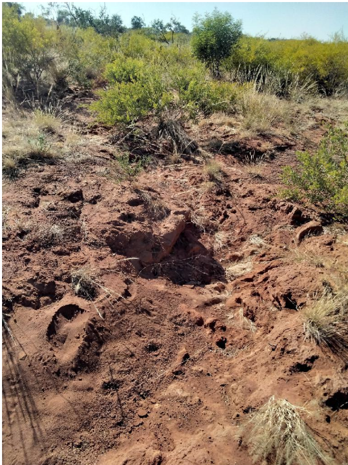
Figure 18. Compromised berm resulting in moderate erosion at KP 25
