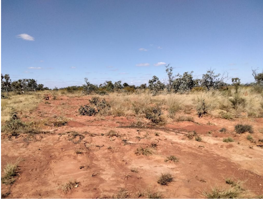
Figure 18. Compromised berm resulting in moderate erosion at KP 25
