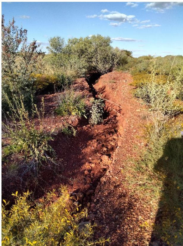
Figure 13. Moderate gully erosion up to 300mm deep at KP 29.3
