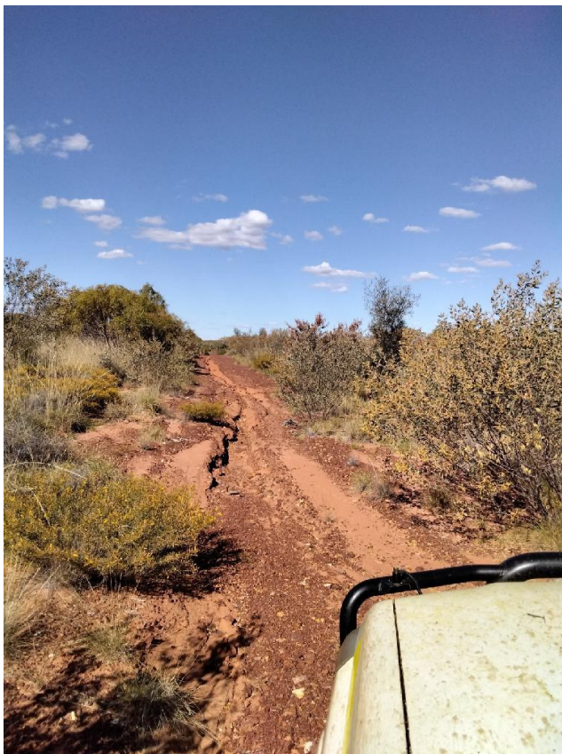
Figure 16. Significant rill erosion up to 500mm deep for approximately 200m at KP 272.6
