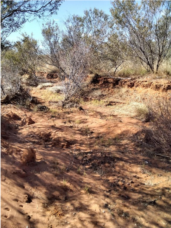
Figure 11. Significant erosion with over 700mm deep gully erosion KP 267.5
