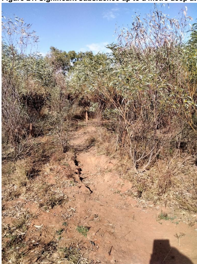
Figure 21. Significant subsidence up to a metre deep at KP 25 where runoff follows the pipeline trench.
